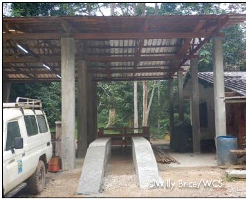
Extension of the mechanical workshop completed.
